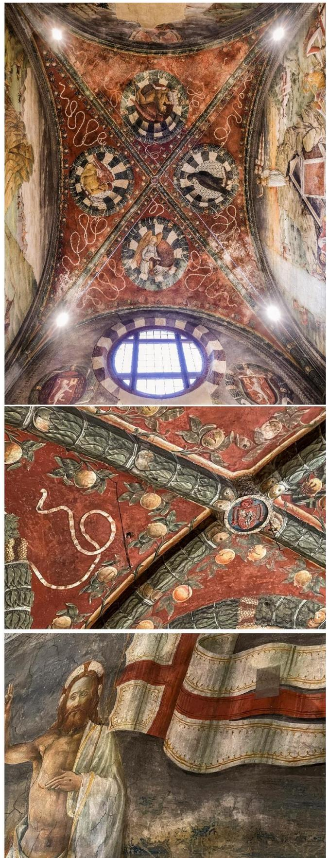
Figure 3. Intrados of the vault of the Castiglioni Chapel and evident deterioration and criticalities of the wall frescoes.
