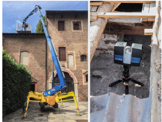
Fig. 5 Elevator platform used to access the extrados of the Chapel vault.
