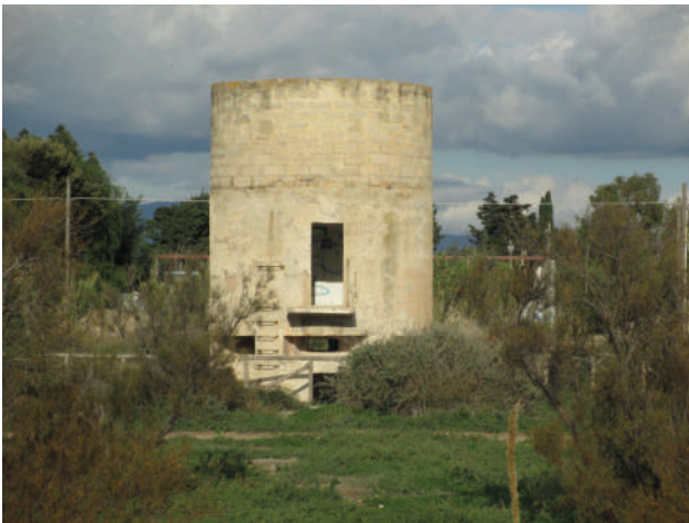
Fig.9. Bunker as a cylindrical water tank - sector 3
