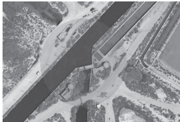
Fig. 15. Bunker located in the sector 2
