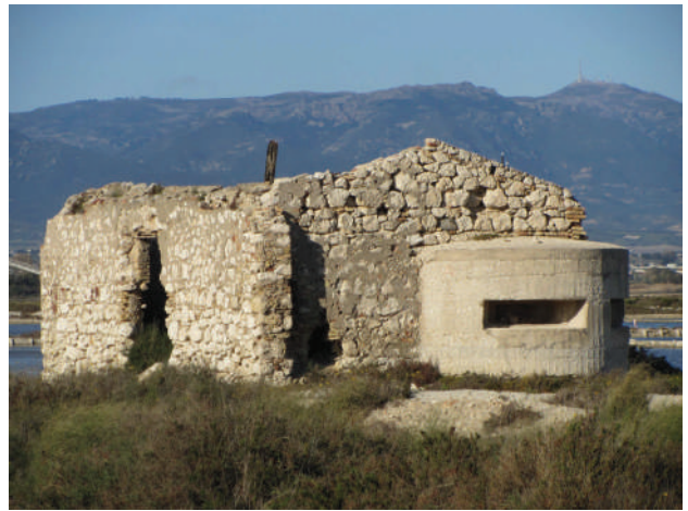
Fig.12. Bunker incorporated in a building - sector 1
