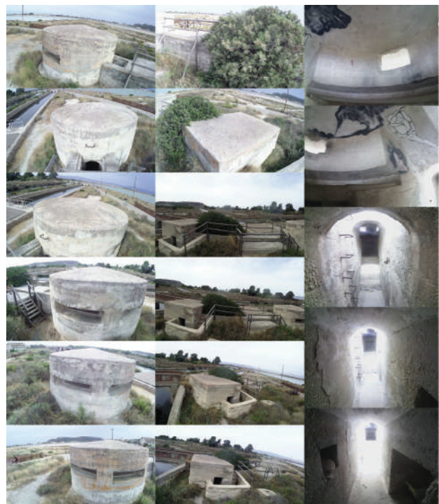
Fig. 16. Photographic survey– sector2
