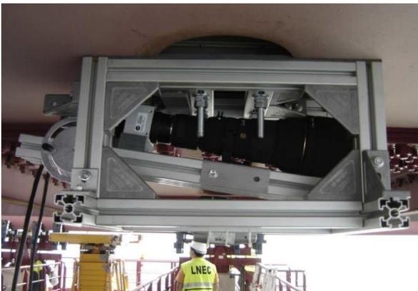
Figure 3. Digital camera installed in the stiffness girder.
