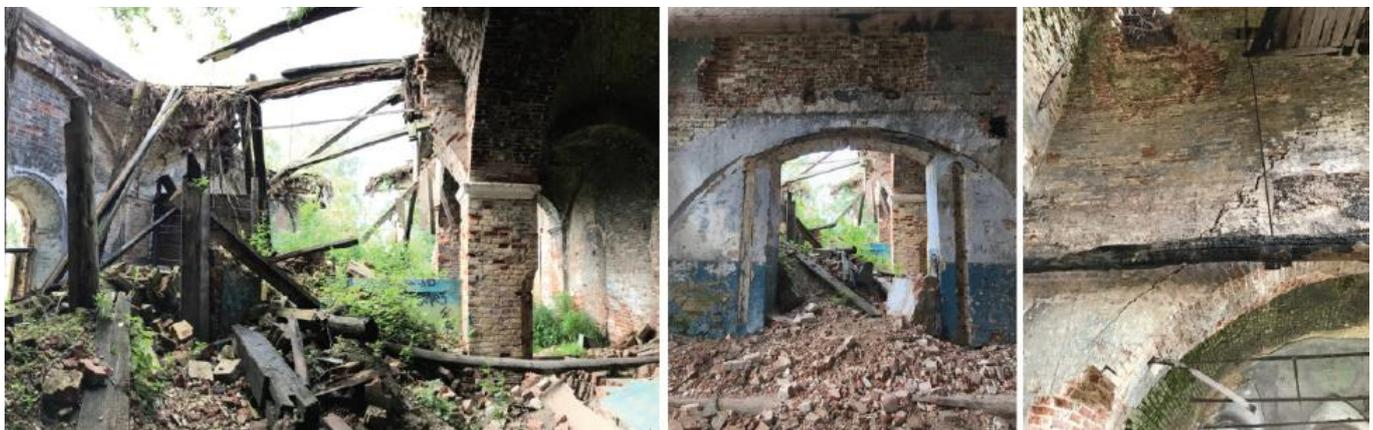
Figure 2. The state of neglect and the lack of conservation present critical situations of widespread instability among the masonry systems, clearly exposing the structure to the damage affecting its elements. Robustness instabilities in the structural complex of the Church of the Transfiguration, Pyskor, defining the increasing frameworks of damage that will destroy these buildings without specific lines of intervention.
