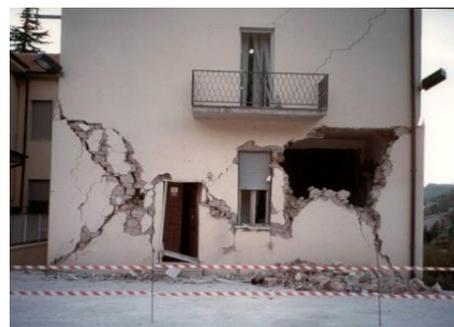
Figure 8. Damage that occurs in piers during a seismic event.
