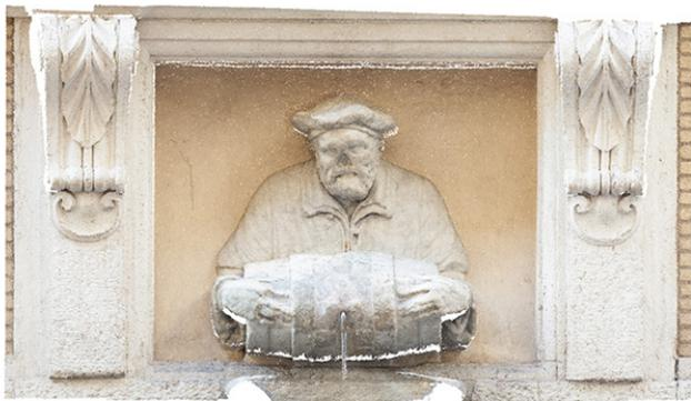
Figure 2. Point cloud of the Facchino's historical fountain in Rome generated with an image-based system. RGB values are taken directly from the camera sensor. The cloud is made up of unstructured data.
