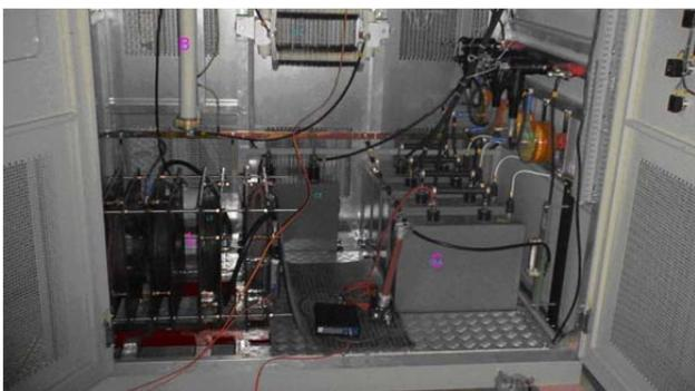
Figure 4. Measurement system in a DC side filter cabinet in a 3 kV DC traction substation (C- capacitance, B- fuse).
