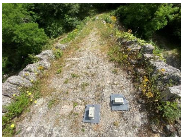
Figure 5. Couple of mechanical seismometers positioned on the roadway of the Roman bridge.
