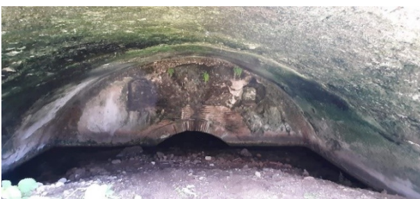
Figure 2. Frontal photo of the nearby nymphaeum , with the clear presence of brackish water on the lining.
