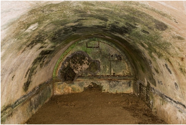
Figure 1. Frontal photo of room SB-E0-R07, taken from the entrance. Biodegradation is evident, particularly on the back wall and on the ceiling.
