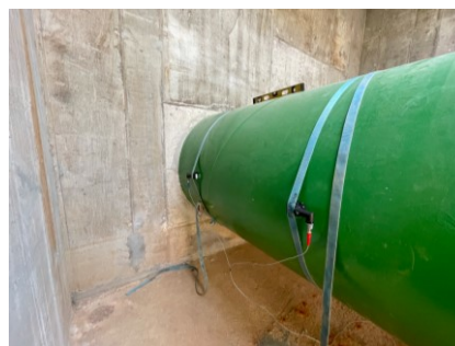
Figure 3. Flowmeter ultrasonic sensors installed in the pipe.
