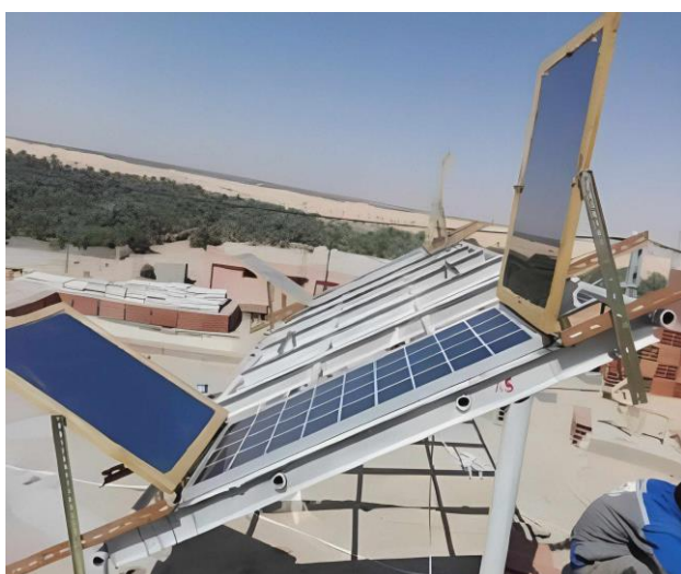
Figure 2. Installation of reflectors on the PV module
