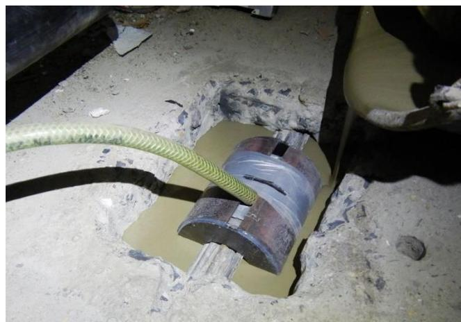
Figure 3. The fully equipped ME sensor installed on the prestressed cable, consequent filling of the created opening by the special grout
